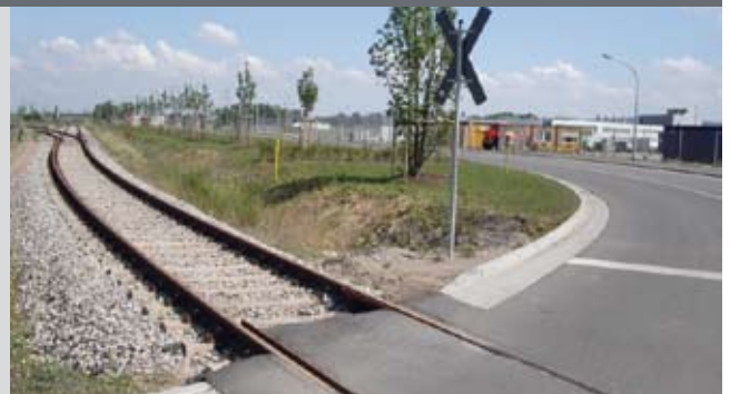
Rail traffic system at Kölleda-Kiebitzhöhe Industrial Park
