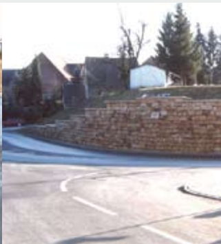
Retaining wall in the cross-town link in Utenbach (L: 75m, W: 1.14m, max. height: 3.26m)
