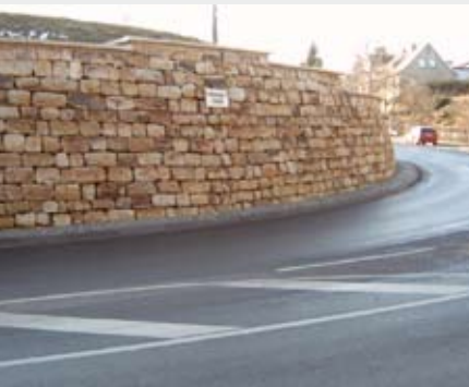
Retaining wall in the cross-town link in Utenbach (L: 75m, W: 1.14m, max. height: 3.26m)
