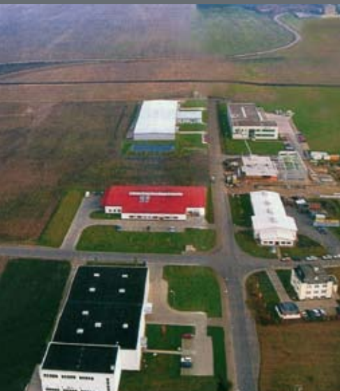
Development of industrial park Kölleda Kiebitzhöhe
