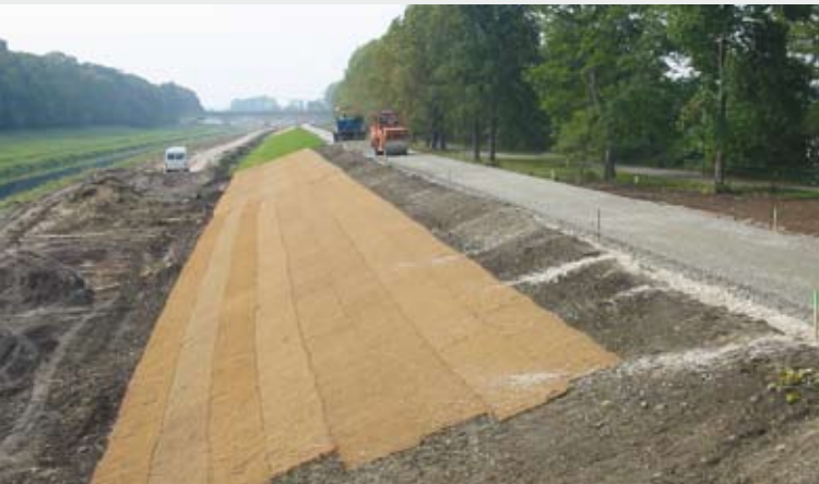
Repair, 1st phase of construction
