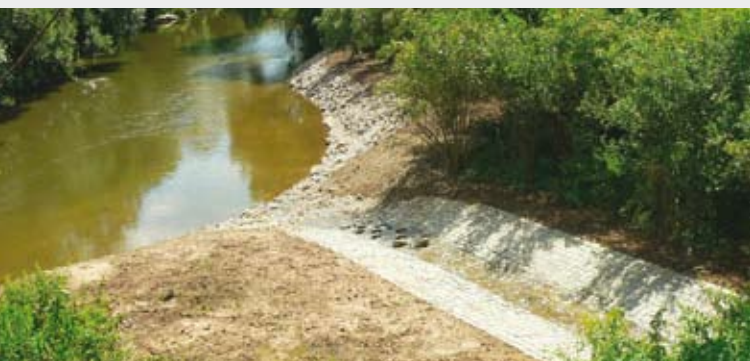
Shoreline stabilization and channel „Am Utmich“
