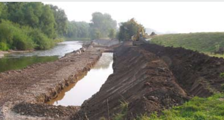
Construction work on dike break
